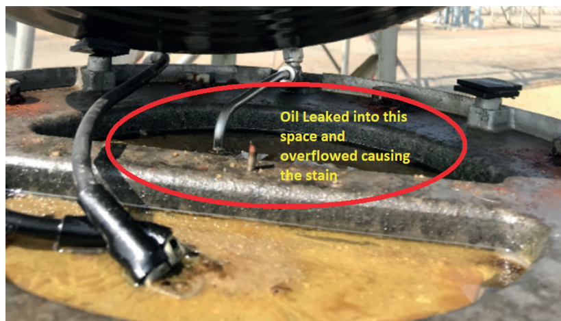
Figure 11: Oil overflow due to puncture on top of C1-B1 section
