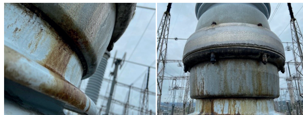
Figure 6: CVT-2 as found during visual inspection
