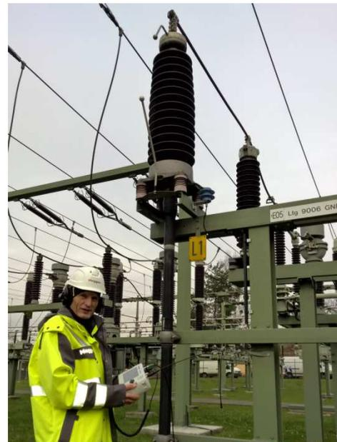
**Figure 12 onsite UHF measurement**
